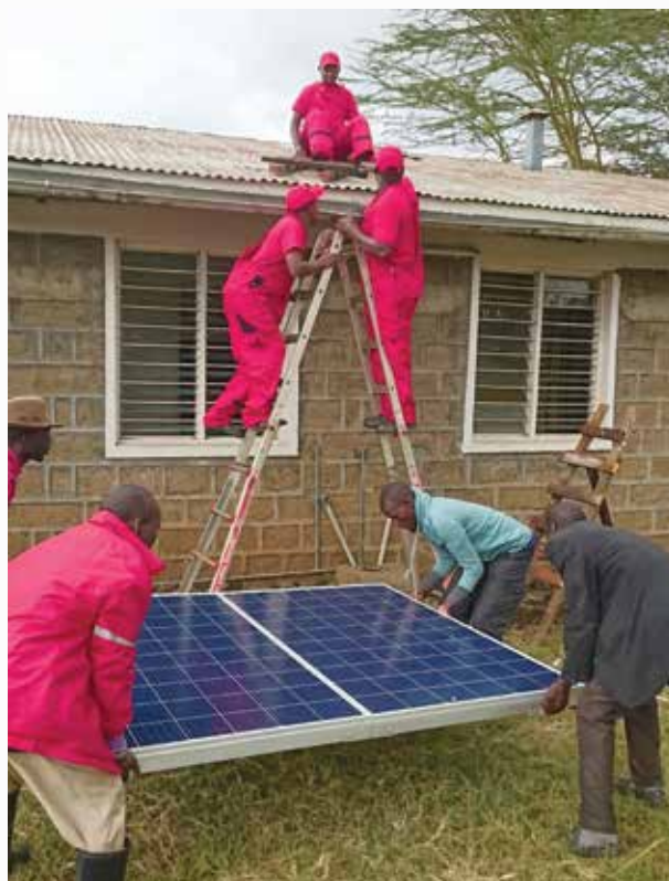
Installation of solar panel for Solarchill fridge.
